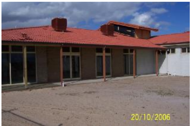
Extended veranda, and new garden entrance doors
