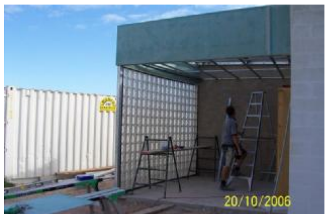
New entrance, looking towards beach
