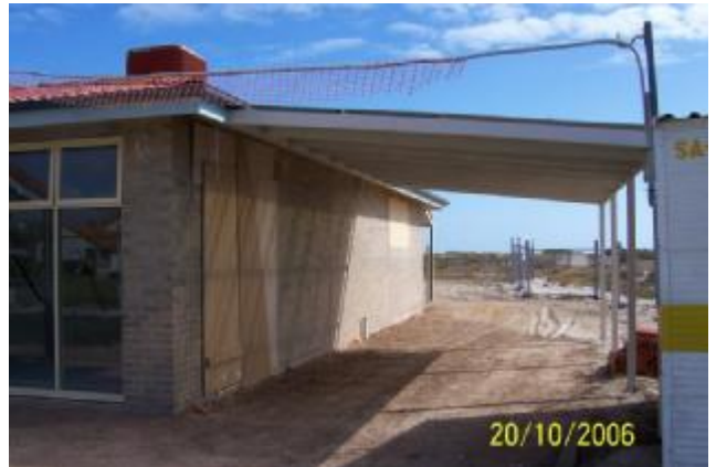
Pergola over Members Area, outside Training Room
